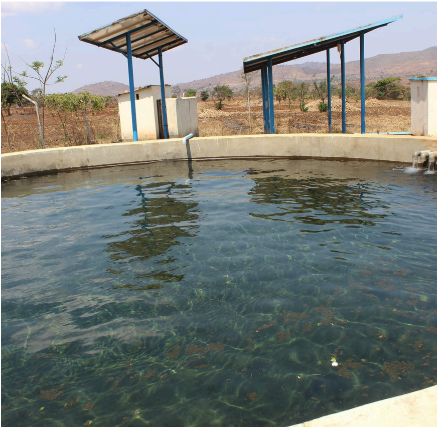
Picture:Tatolonga Irrigation scheme in Dzaleka
