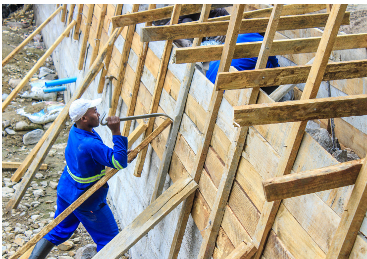
Picture: Construction of a sanddam wall
