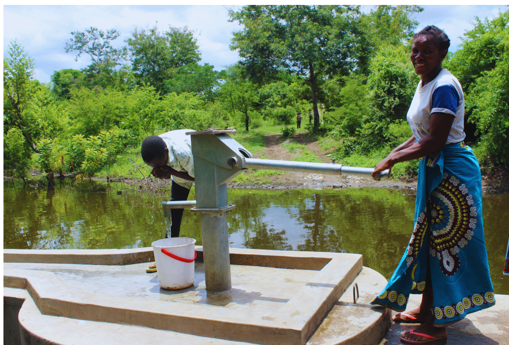
Picture: Accessing water from the sand dam shallow well handpump in GVH Nyanthumbi in Nsanje.
