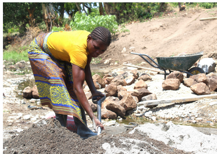
Picture: Siteliya mixing cement during the construction of a sanddam
